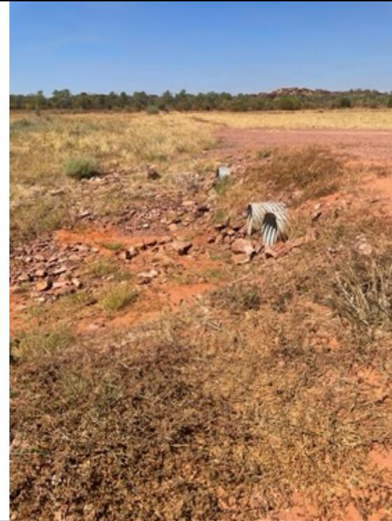
Figure 34: Existing culvert at wpt KCC15
